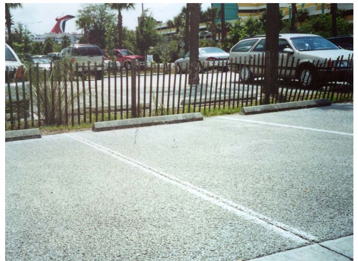
Figure 3-58 Typical Porous Concrete System Applications (Knox Co., TN, 2008)
