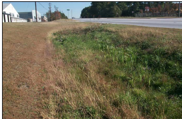
Figure 3-22 Enhanced Swale Example
