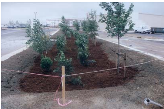
Newly Constructed Bioretention Area
