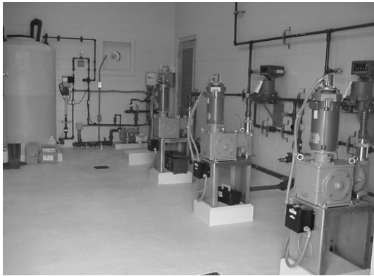
Figure 3-45 Alum Treatment System and Injection Equipment
