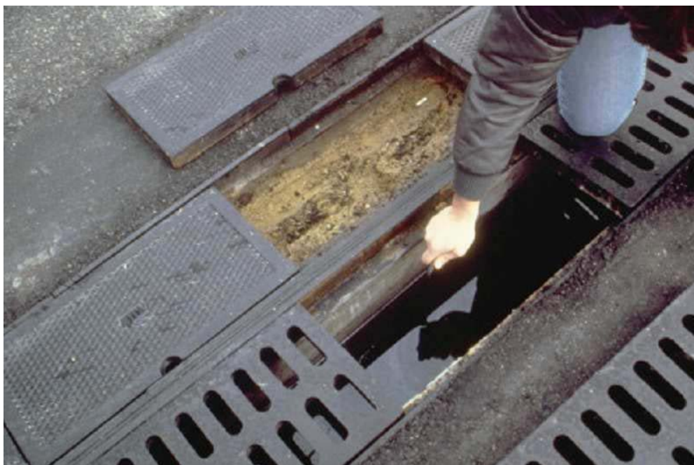
Figure 3-46 Example of an Underground Sand Filter
