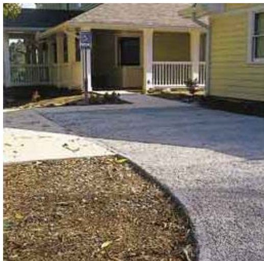
Figure 3-58 Typical Porous Concrete System Applications (Knox Co., TN, 2008)
